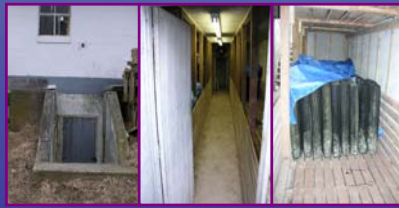
Fig. 4. A typical seed pit is a root cellar, insulated at least in part by earth, with a cement floor and wooden railings, and bags of seed covered under a tarp.
